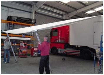
It is recommended that fixing pegs are used to anchor the corner posts into position. The two corners of the front frame should now be tethered to the ground, to help keep the frame in position. This will also stop the roof panels from lifting the frame in windy conditions.
