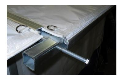
Rotate the tension beams and place over the tension brackets in the end of the roof rail. **Do not** tighten the bolts at this point. Repeat this for each bay. Tighten the bolts once all roofs are fitted.
